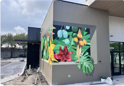
A Window In exterior Aventura, FL
